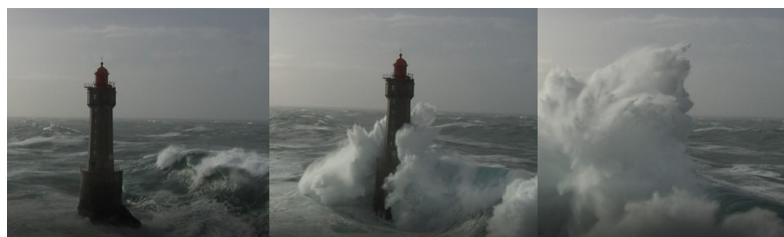
Figure 1.5 – Images of a breaking wave impacting the La Jument lighthouse, situated at the South-West of Ushant ©Air Vide et Eau
