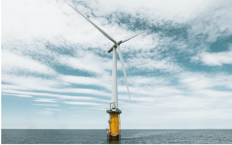
Figure 1.3 – The 2.3 MW SPAR-type prototype Zefyros. Source: Metcentre .
