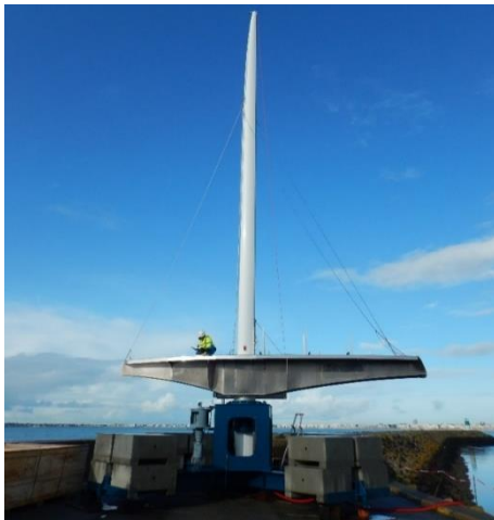
Figure 14 Balestron rig full view.
