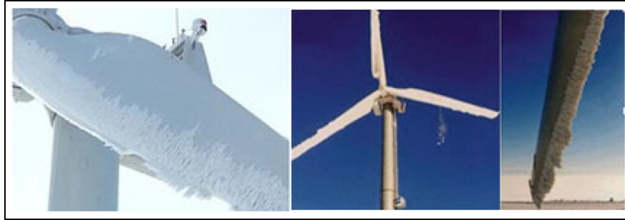
Figure 1. Impact of icing on wind turbines.
