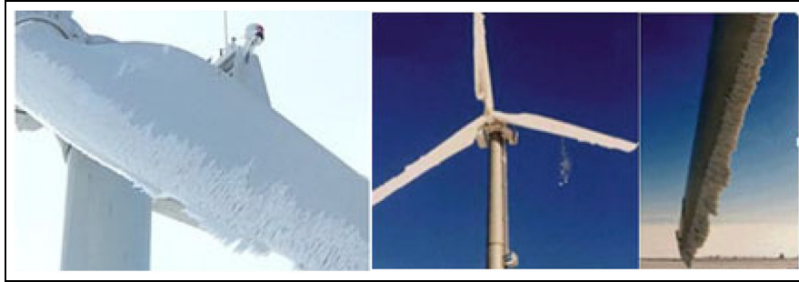
Figure 1. Impact of icing on wind turbines.
