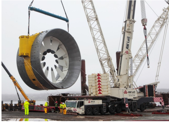
(a) tidal turbine installation
